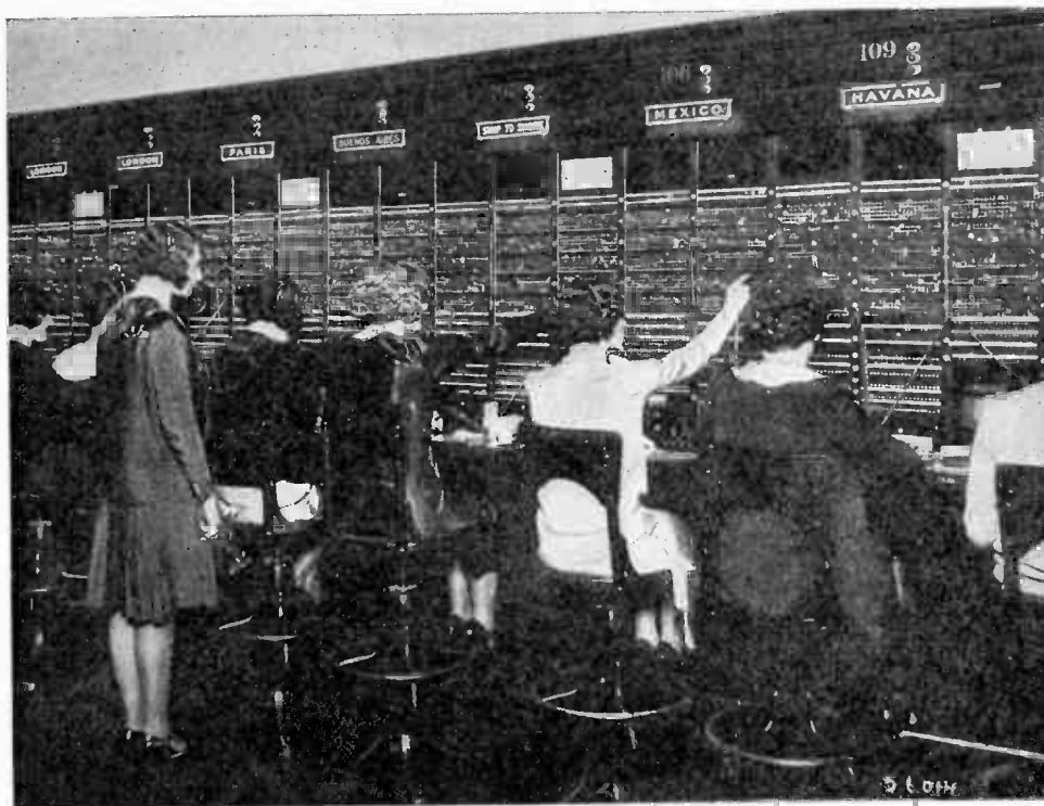
The heart of an international communication system: the foreign service switchboard in the long-distance office of the A. T. & T., at 24 Walker Street, New York City, where calls to Great Britain, France, the Argentine, Mexico, Cuba and ships at sea are handled.
